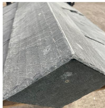
Screw the block end into position through the holes and into the batten using the three RidgeFix 60mm screws provided.
