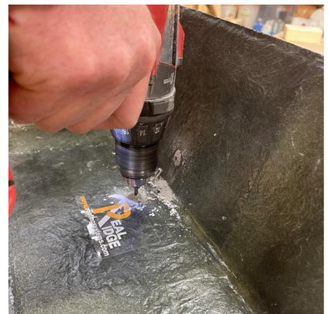
3. Use a 10mm masonry bit to form a 5mm countersink on the outer surface, so that the screw fits flush and the washer seats when installed.
