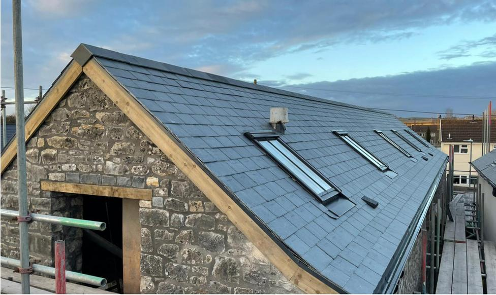
Classic Dry RealRidge Slate is an all-in-one ridge tile system made from natural slate. Its patent pending, interlocking fixing system means it is very easy to install, but watertight whilst allowing ventilation. Natural slate and invisible fixings means RealRidge is the best looking ridge available with a seamless fit on the roof.
