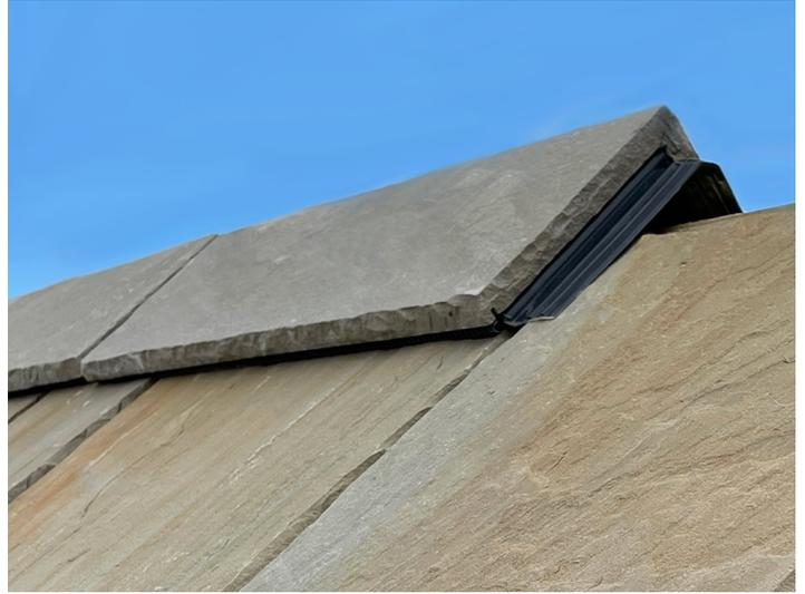
The first ridge should always be double fixed into position using 2 RidgeFix stainless steel screws with nitrile washers -
