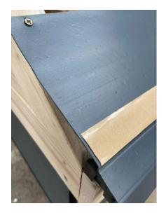
Install an eaves protection system (EPS) or starter trim directly on top of the rafter so that it sits over the fascia directed into the gutter. Securely fix through the top section of the EPS to the rafters. Lengths of the EPS/ starter trim should be lap joined on top of a supporting rafter.
