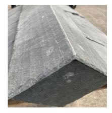
Screw the block end into position through the holes and into the batten using the three RidgeFix 60mm screws provided.
