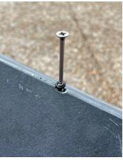
Place over the two connectors in the gap and double fix with 2 x 100mm RidgeFix screws (supplied).
