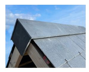
The first ridge tile or block / hip end should always be double fixed into position using 2 RidgeFix stainless steel screws with nitrile washers -
