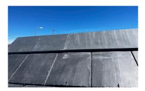
Continue along the ridge, fixing each ridge tile with 2 x screws.
