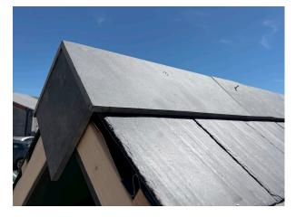
If not using a block / hip end, starting from one side, the built in GRP RealRidge connector faces inward so that the next RealRidge sits over the top of the GRP strip.
